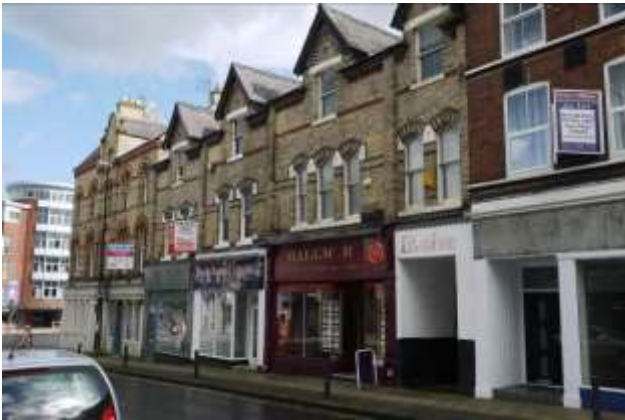
Late Victorian buildings in commercial and retail use on the lower Downs with some poor ground floor frontage alterations
