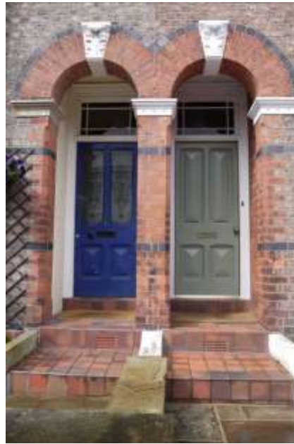
Original doors on New Street
