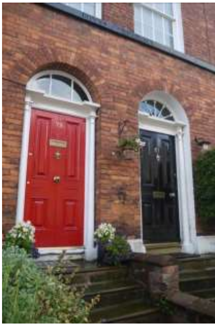
Original doors on New Street
