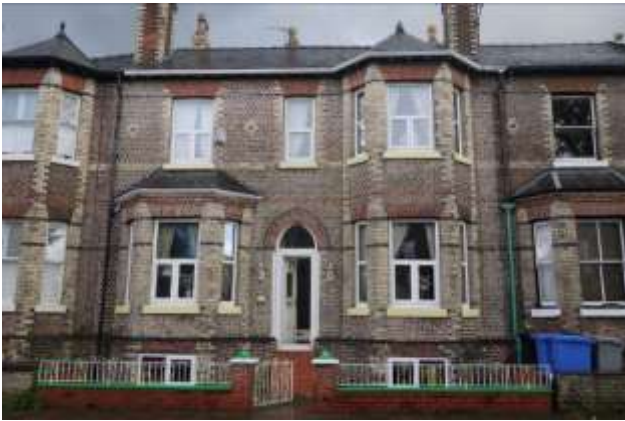
Substantial Victorian terraces, many have suffered from inappropriate replacement of features such as windows, doors and boundary walls
