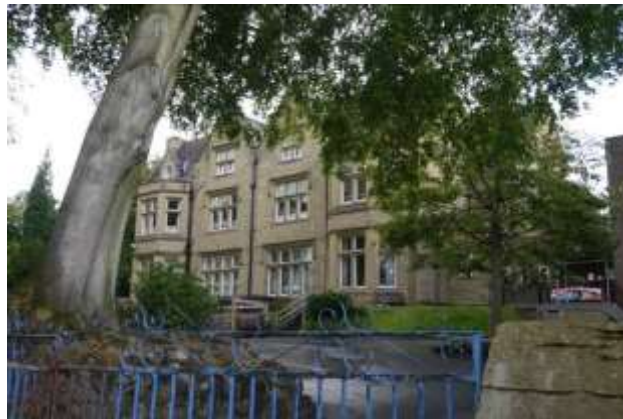
Rusticated stone is used in the Conservation Area on the larger buildings. Bowdon Preparatory School
