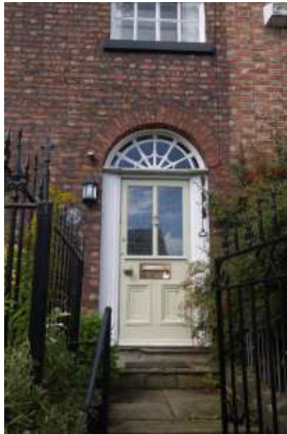
Original fanlight, bell pull and railings on No. 42 The Downs. The door is a slightly later replacement with stained glass
