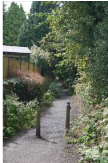
The Narrows, note the inappropriate timber fencing
