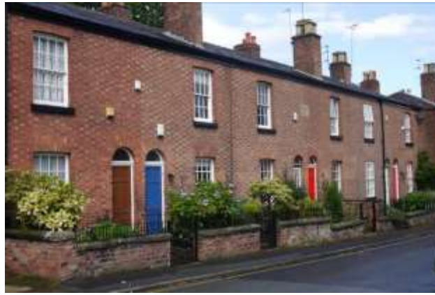
Simple classical terraced houses with round arched doors, 8 over 8 sash windows and Flemish bond brickwork at 46 New Street
