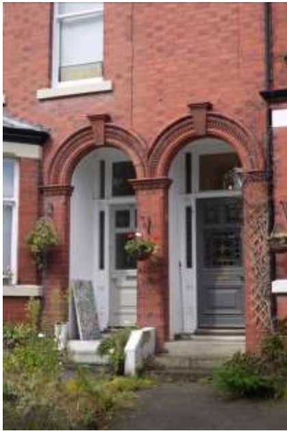
Original doors on The Downs with timber panels and stained glass
