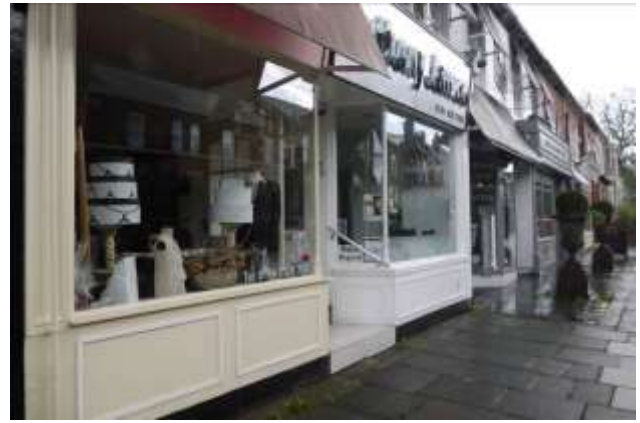
Original shop fronts with stall risers, slender glazing bars and panelling. The fascias are not appropriate
