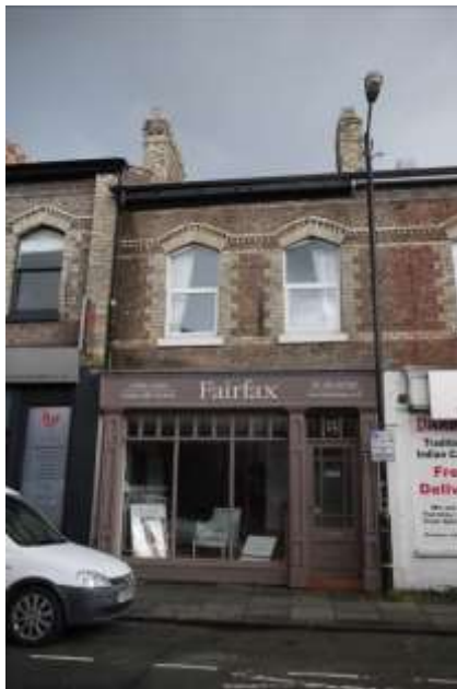
Traditional replacement shop front on Oxford Street
