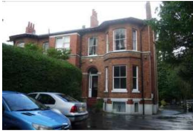
Italianate features such as deep bracketed eaves and double height bay windows can be seen on Hale Road. Note the converted basement
