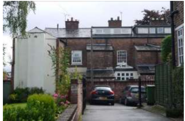
Rear elevation showing rendered outriggers, ground floor extensions and converted attic spaces with additional windows
