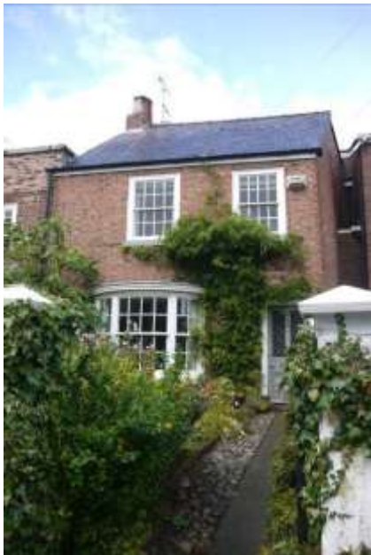
Flemish bond brickwork, slate roofs, doors bow windows, original timber sashes and mature planting
