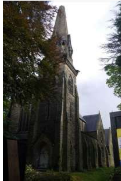
Redundant church on Delamer Road prior to work starting on a residential scheme
