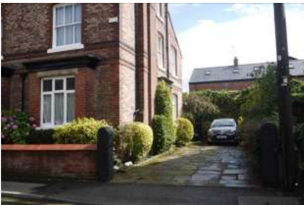
Gateposts have been painted and possibly front widened to create a driveway
