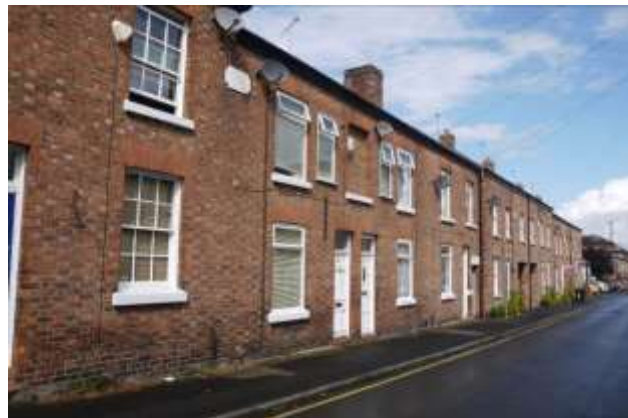
Simple terraces on New Street harmed by inappropriate style sash doors, uPVC windows and intrusive satellite dishes
