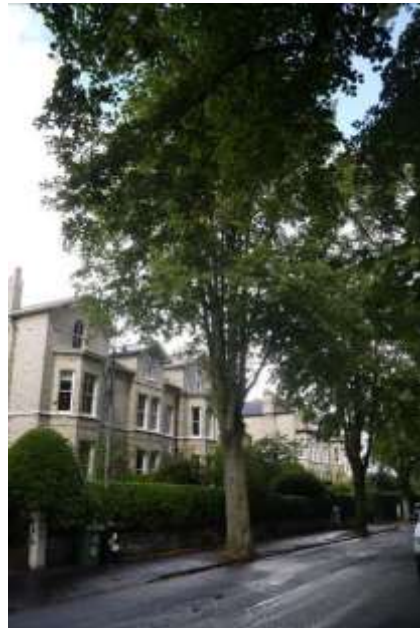
Example of the cream 'Bowdon' brick buildings on Delamer Road
