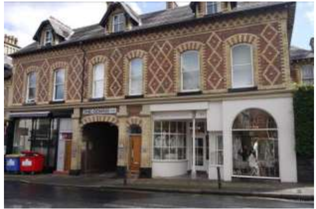
Shop fronts along the lower Downs
