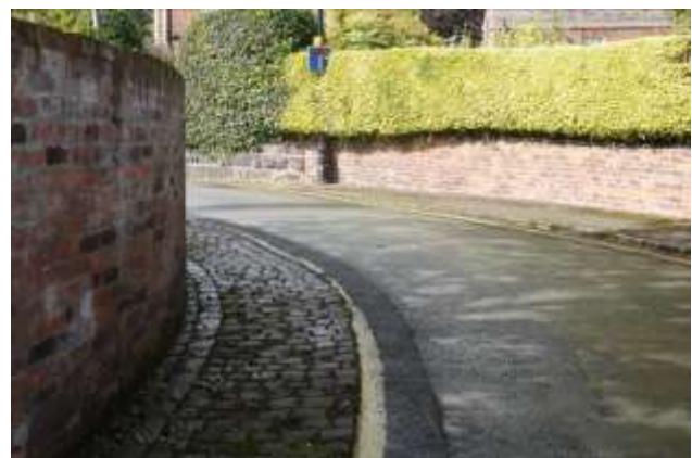
Traditional stone setts and more modern surfaces sit side by side on Lyme Grove
